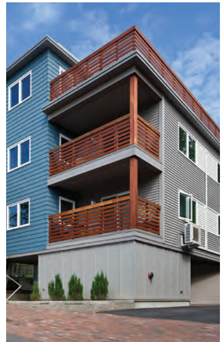
From top down: Solar panels at Aikido of Maine, installed by ReVision Energy // LEED Gold-certified Portland International Jetport // Net Zero apartment building at 62 Cumberland Ave., designed by Kaplan Thompson Architects; solar photovoltaic and hot water systems are the sole sources of energy for this super-insulated building
